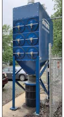
Avani Model Six-Cartridge Dust Collector
