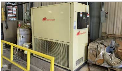
Ingersoll Rand Refrigerated Air Dryer
