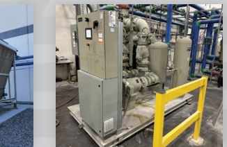
Complete Chiller System w/ (2) 160 Ton Trane Chillers, Towers, Tanks and Pumps
