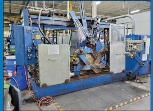
(2) 150 KW Tocco Induction Static AC-DC-AC Frequency Converter Using Nominal 480 VAC, 3-Phase, 50/60 HZ Power Supply
