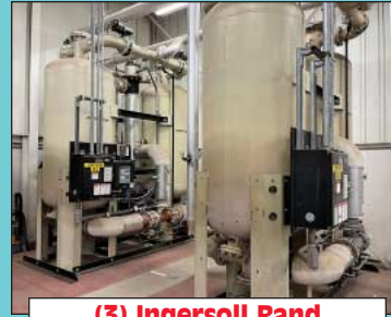
(3) Ingersoll Rand Desiccant Air Dryers
