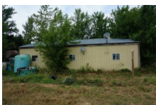
36' x 46' Shop w/ concrete floor
