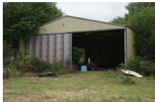
40' x 72' Machine Shed
