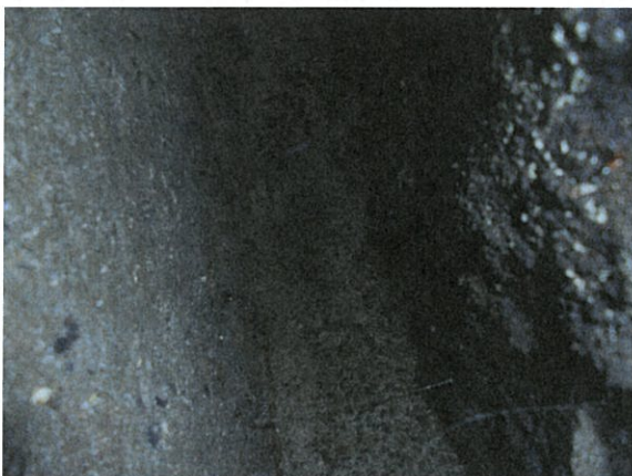
Roof of tank
