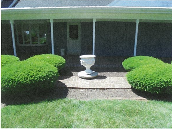
Location of first septic tank
