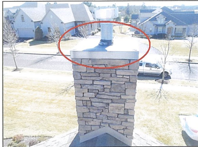
3.0 Item 10(Picture) Chimney cap was in good condition
