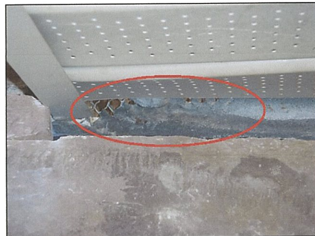
3.0 Item 14(Picture) Wire lath and OSB visible under soffit on chimney
