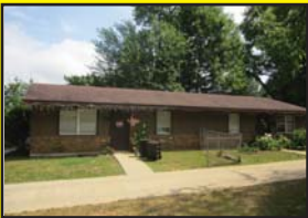
#1. NICE BRICK/ SIDING DUPLEX & LOT 422 A & B HARGROVE ST. ATHENS, AL. 35611
