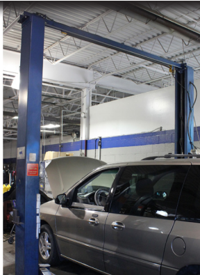
#258 - 273 Challenger, Forward, & Workhorse Automotive Lifts
