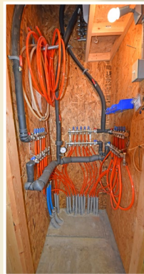
PIPING FOR HEATED FLOORING IN POLE BARN
