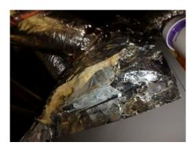
24. Loose/damaged insulation was noted on the HVAC ducts at the HVAC unit. Repair as needed.
