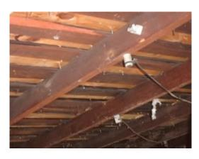
22. Knob and tube wiring was visible in the attic. The knob and tube wiring was not accessible due to no flooring. Knob and tube wiring is considered to be outdated and is a fire hazard. Knob and tub wiring should be removed/replaced by a licensed electrical contractor to maintain safety.
