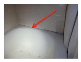
12. The gaps in the downstairs bathroom shower stall should be sealed to avoid moisture intrusion into the flooring and walls.
