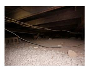
27. No vapor barrier was noted on areas of the crawlspace floor. A continuous vapor barrier is recommended to reduce condensation buildup in the crawlspace.
