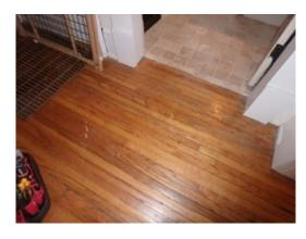
7. Soft flooring was noted in the hallway. Further investigation is recommended by a qualified professional with corrections made as needed.
