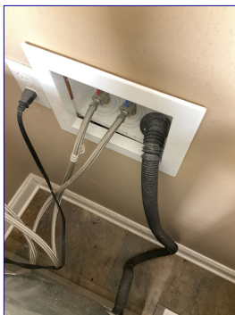
Laundry, washer hook-up view
