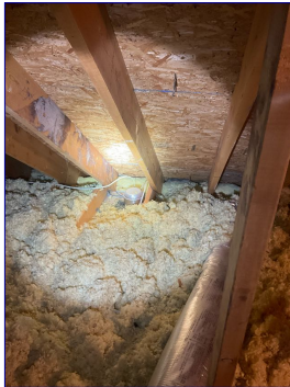
Missing baffles
