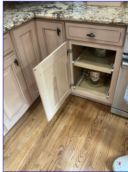
Loose cabinet hinges
