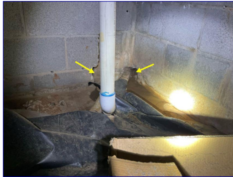
Wall penetrations need to be sealed
