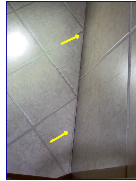
Needs caulking/sealing
