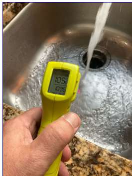
Hot water temp
