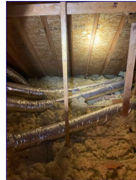
Missing baffles
