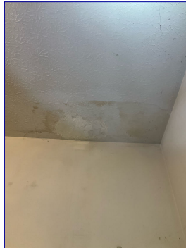
Moisture stains/damage
