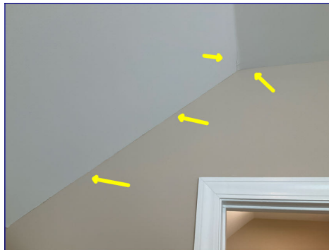
Settling cracks
